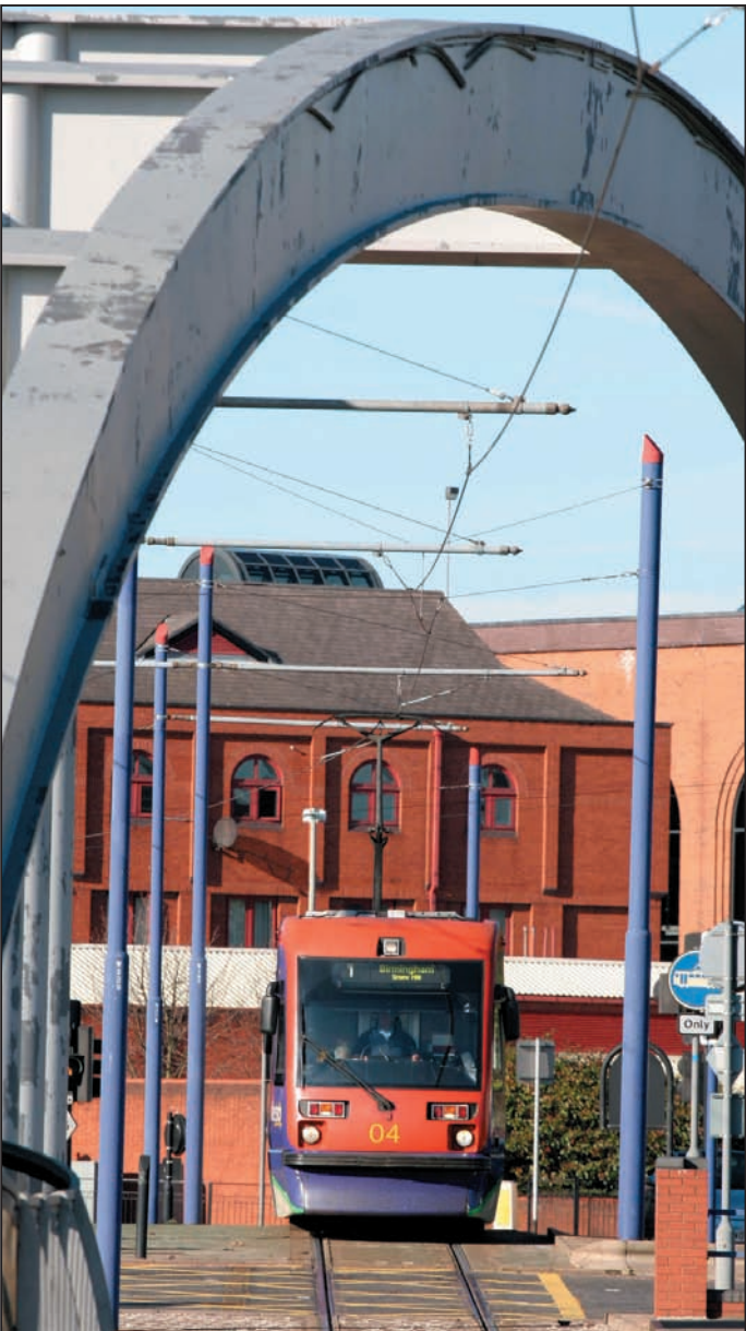
The bridge before work began
